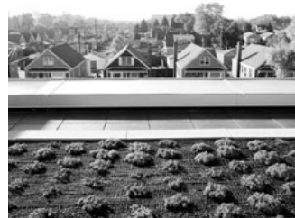
A drought-resistant/insulating roof: for teaching and energy efficiency: Tarkington ES, Chicago
